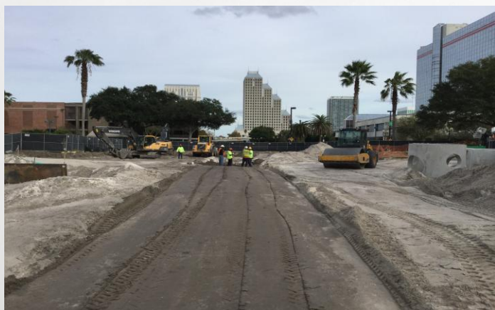
Livingston Street: Crews installing sanitary line up to manhole
