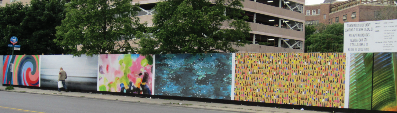
Artist-designed Construction Fence, CAMBA Gardens Apartment Project, Brooklyn, New York.
