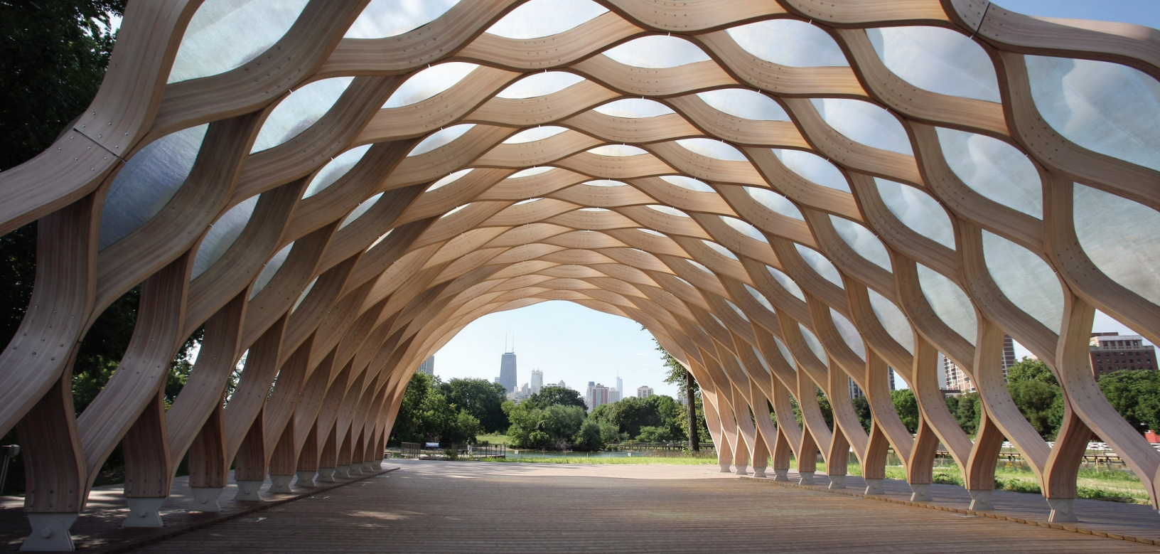
Artworks along pathways: Archway , Gang Architects, Chicago, Illinois.
