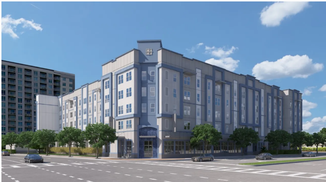
The redesigned Beacon at Creative Village will be five stories and will have 115 apartments. (Rendering by Slocum Platts)
